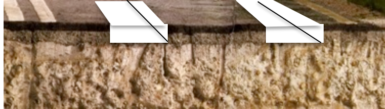
STAGE One : Grooving road 200mm x 400mm
